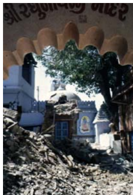
Damaged Cultural Heritage by Earthquake (Gujarat, 2001)
